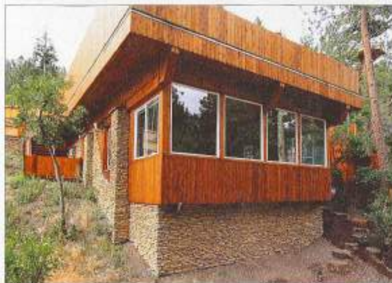
A-FRAME NO MORE - You wouldn't know it from this photo, but this retreat was an A-frame before a devastating fire burned it to the foundation. Instead of restoring the A-frame, the owners rebuilt the cabin as a bungalow with a rooftop garden.
